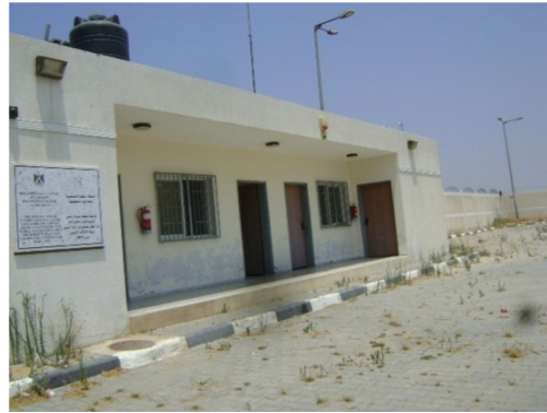
Electrical supply station in BLWWTP
