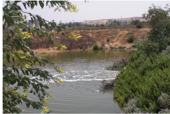
Pond # 4 (aeration pond)
